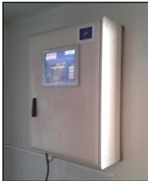
Programmable Logic Controller (PLC)
